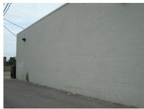
The exterior walls are concrete block. The front elevation has a brick veneer.
