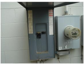
The grocery store is equipped with a 3000-amp 208v/120v 3 phase four wire system. Dominos has a 200-amp 208/120v 3 phase 4 wire; The vacant store has a 100 amp 208/120v 3 phase 4 wire and a 100 amp 208v/120v 3 phase 4 wire house panel is located at the rear of the building.
