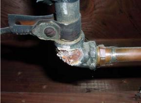
Some corrosion was noted between steel and copper piping. A dielectric connector is required to separate the metals. **Water Pressure:**
