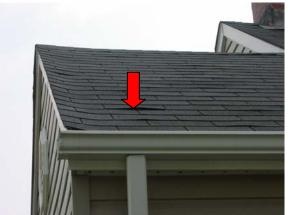
Some nail pops were observed due to improper nailing. The garage roof needs to be replaced.
