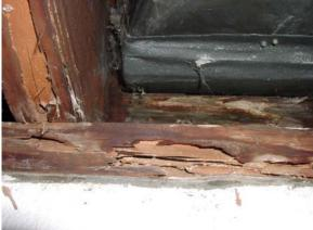
Some minor termite damage was observed at the northwest corner near the basement window. Repairs are considered discretionary.
